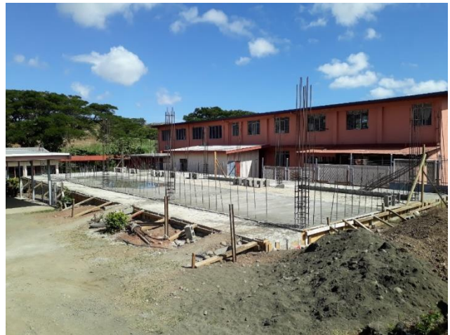
Penang Sangam High classroom project – work under way
