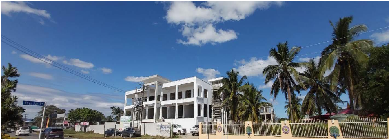
SANGAM CULTURAL COMPLEX NEARING COMPLETION
