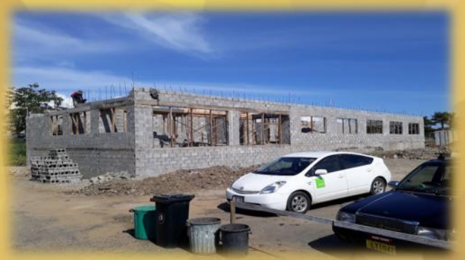
PROGRESS OF WORK AT THE NADI SANGAM TEMPLE VEGETARIAN RESTAURANT
